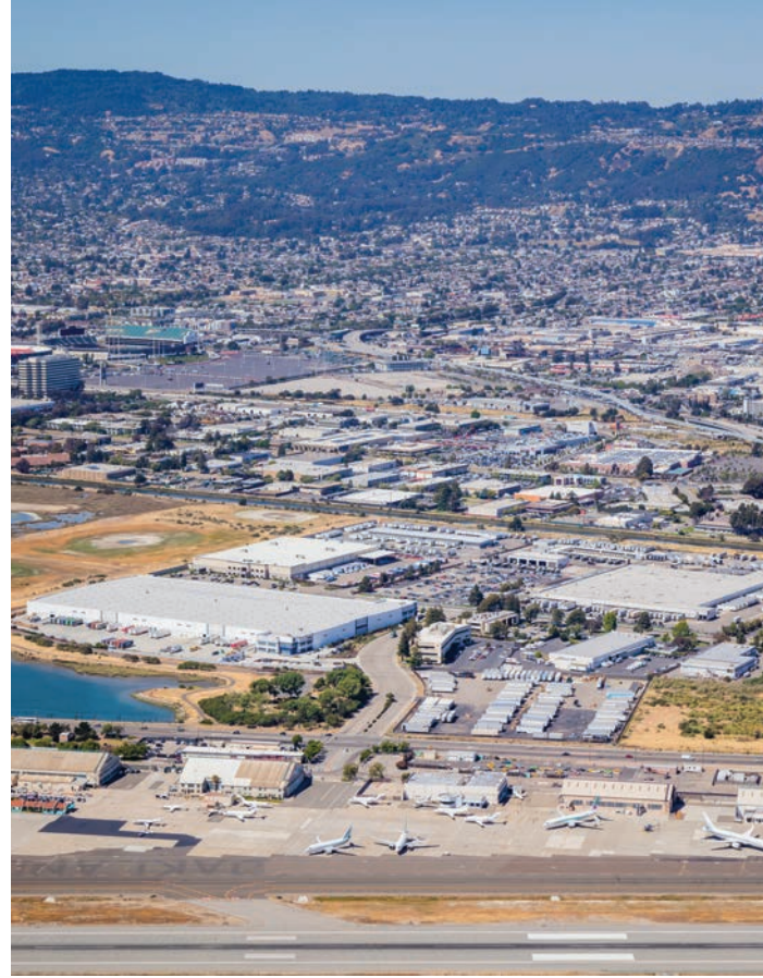
Prologis Oakland 5 INDUSTRIAL | Oakland, CA Prologis Targeted U.S. Logistics Fund
