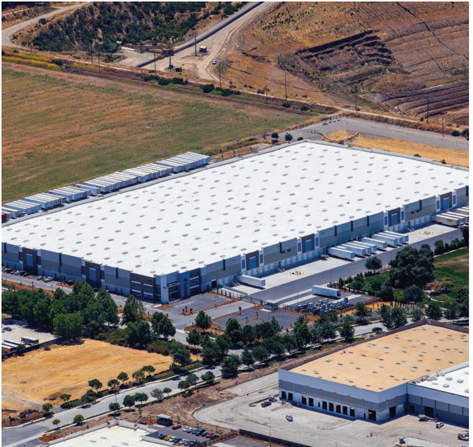
Livermore Distribution Center INDUSTRIAL | Livermore, CA BGO Diversified US Property Fund
